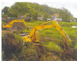
Phumdi removal with excavators
